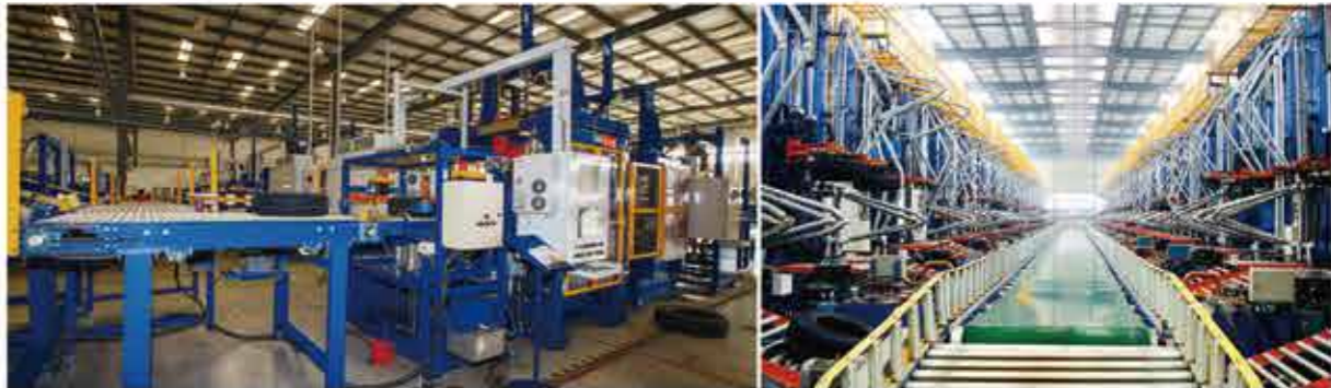
• Automatic tiered warehouse facility curing moulda • Extruder line From Germany Troester
